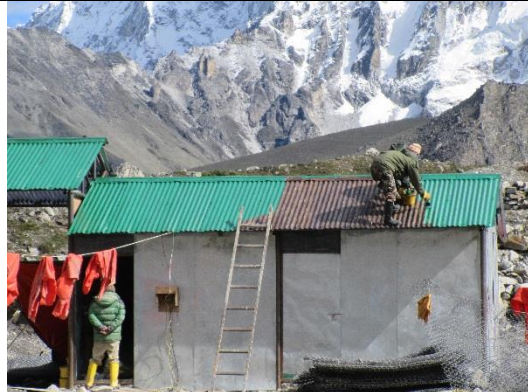
Warehouse roof being painted green as per the SNP guidelines.
