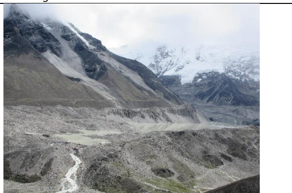
Overview of Imja Lake where lake lowering construction is ongoing.
